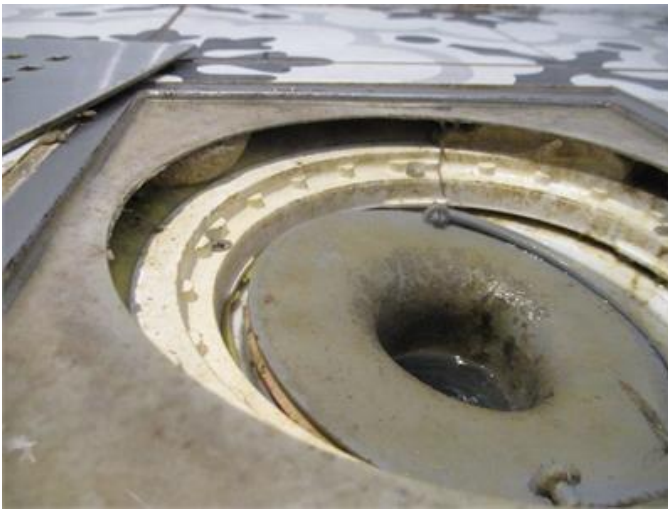
Manschett synd under klämring i badrum.
